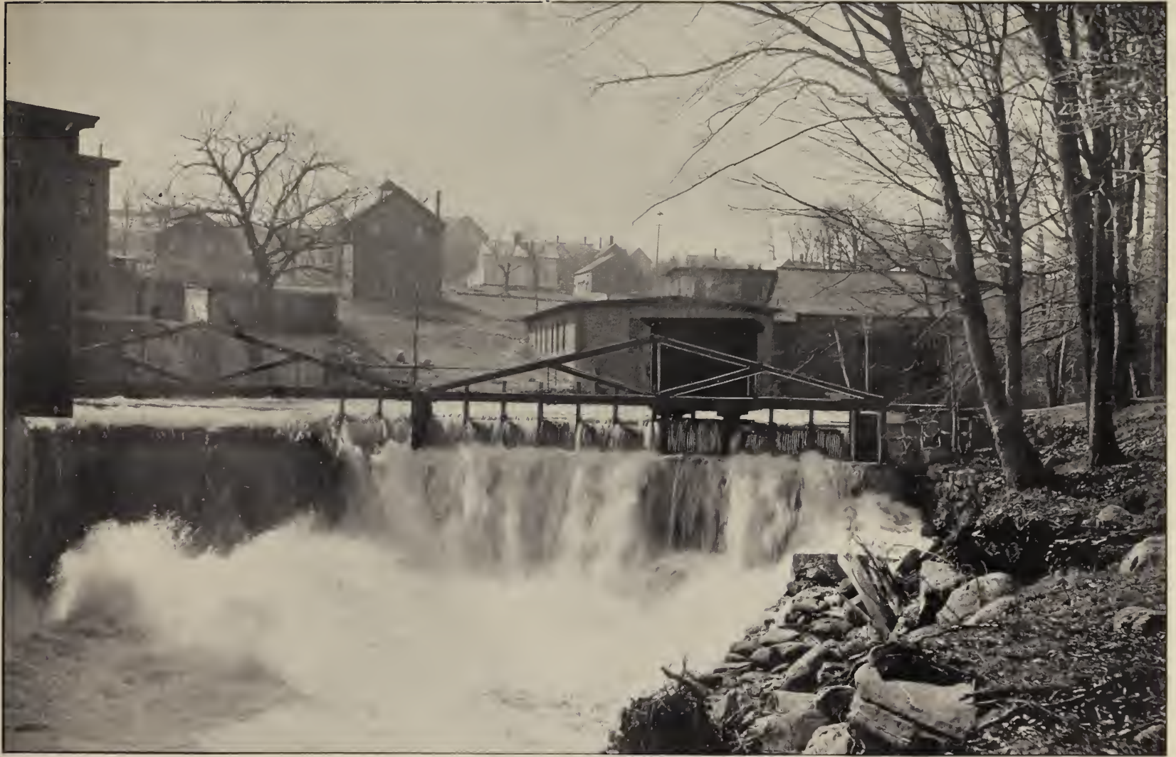
DAM NO. 6, OWNED BY THE S. D. WARREN & CO. PAPER CO.—FALL 17.51 FEET. See Page 35.
